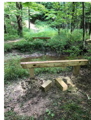
The start of the new bridge.
